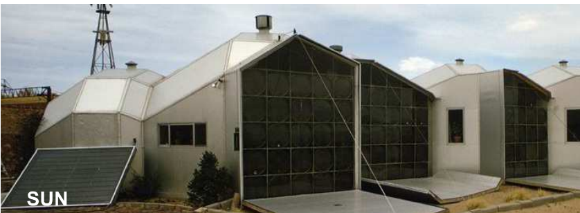
Baer House, Corrales, New Mexico, 1971, solar collectors and windmill waterpump Source: http://www.sorryoutofgas.org/
